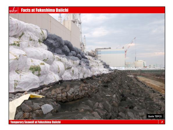
What you see here is temporary newly-constructed seawall to prevent damage by another Tsunami. This wall is 50 feet high above the sea level, while the last tsunami had 40 feet height.
