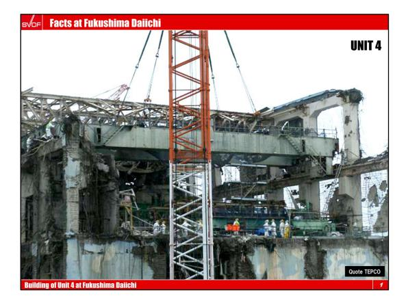
This is the building housing of Unit 4. Spent fuel pool of this unit, which contains 1535 spent fuel rods, has been a big source concern recently. That concern is due to the ever-present danger of another earthquake occurring and causing the water to drain from the pool, which would unleash a nuclear fire. Consequently, efforts have been made to reinforce this building.
