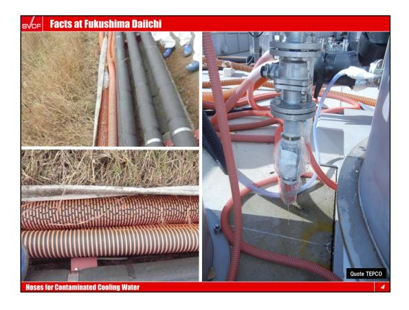
Here, you see hose lines conducting cooling water to nuclear vessels. It should be noted that such a flexible hoses like these are prohibited for use in any plant meant for long term operation. They may be employed only emergency situations, such as fire fighting since such a plastic hoses are weak to weathering.
